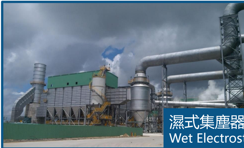
靜電集塵器 ESP Electrostatic Precipitator
